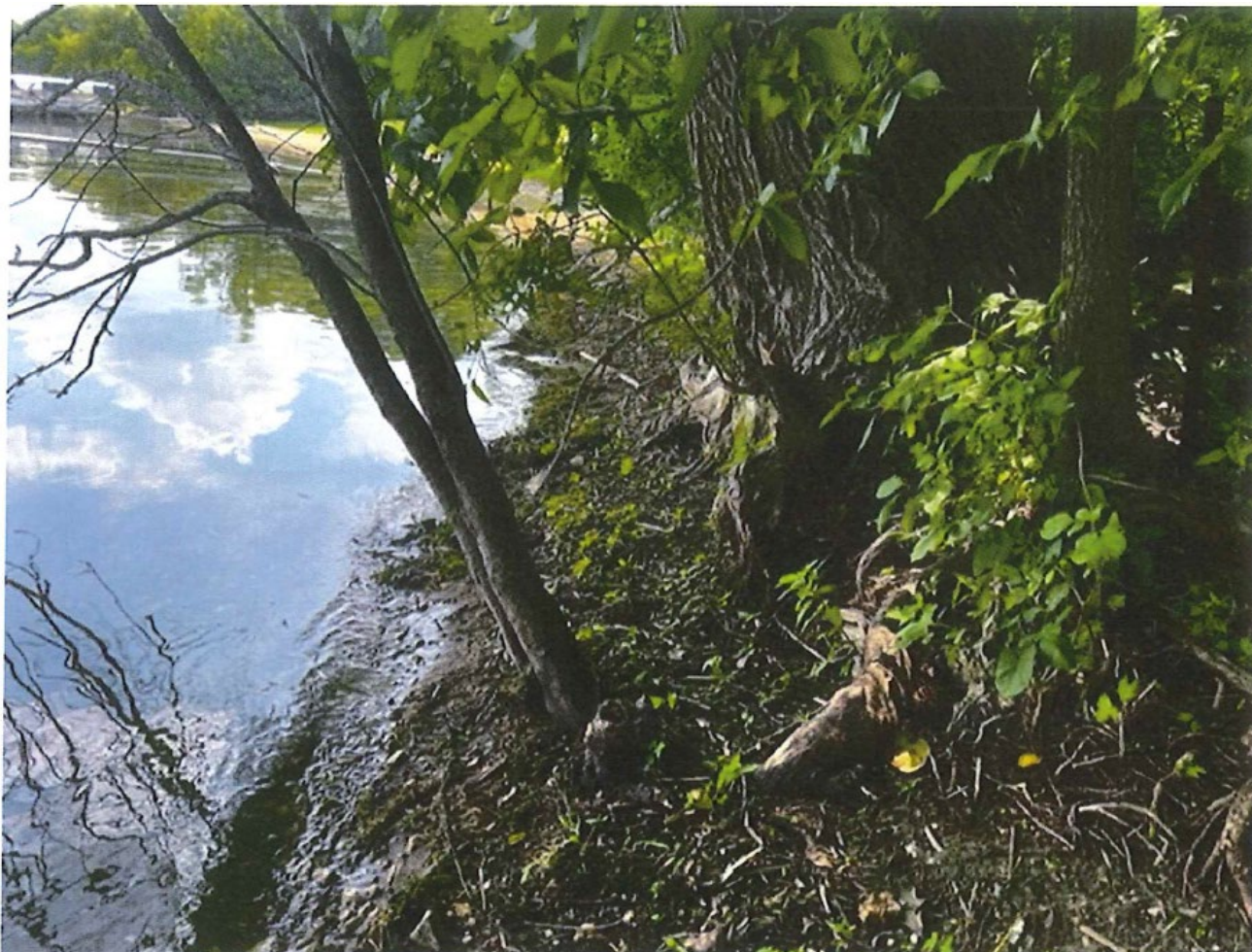
Picture of eroding lakeshore provided by landowner/contractor
