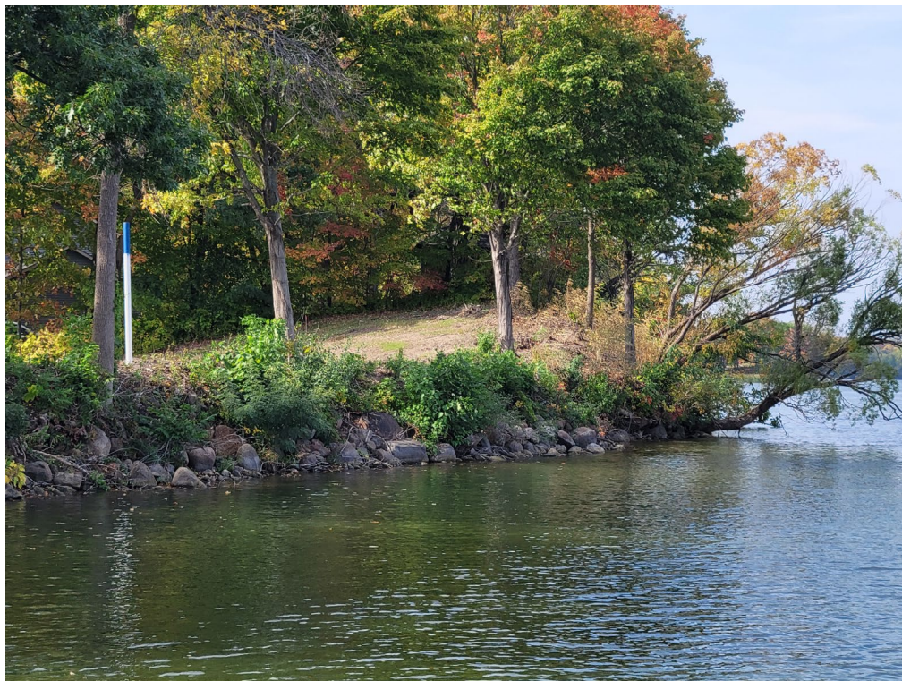
Picture from dock depicting hard armoring and extent of slope on lot 4
