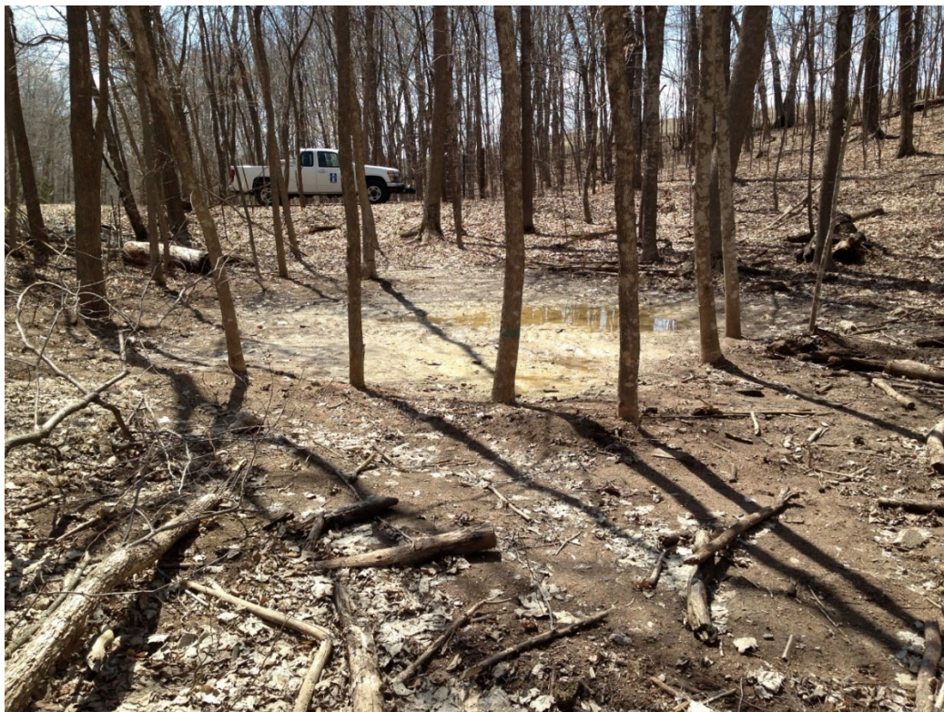
Sediment Deposited from Culvert Outlet.
