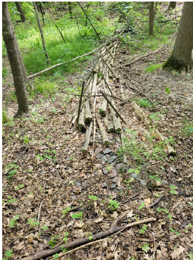
Debris Dams installed to slow the water downstream.
