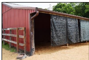
Sturdy roof gutters with downspouts direct clean water away from lot underground to grass waterway.
