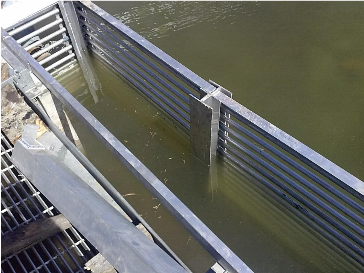
Figure 3. Example of Removable Fish Grate with Horizontal Bars.
